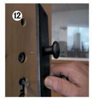
If necessary, cut turnpiece spindle so it reaches halfway through the lock but does not interfere with inside wall of lock cavity. Fit interior piece.
