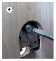
Fasten spinde into position with screw from outside of door.
