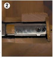
Adjust bevel by loosening screws on top and bottom of lock. Do not remove screws. Once bevel is correctly set, tighten screws and install lock in door.
