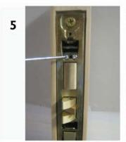
Loosen screw on lock front to allow entry of cylinder.
