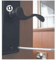
Locate machine screws into threaded posts on outside trim. Use of power-tools is not recommended as they increase chance of stripping screws or scratching trim.
