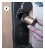
Rotate swing cover and locate cylinder into lock.
