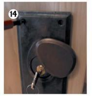
Ensure outside trim is properly positioned then drill pilot holes for wood screws. Secure outside trim with wood screws. Finally, attach screw cover on inside with machine screw provided and attach finished scalp to lock front.
