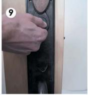
Check operation of lock for both latchbolt and deadbolt retraction.
