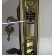
Tighten screw on front of lock to secure cylinder in position.
