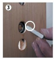
Insert knurled end of spindle into the lock from the inside of the door.
