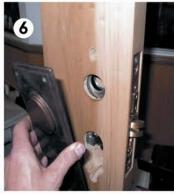
Locate exterior plate but do not secure at this stage.
